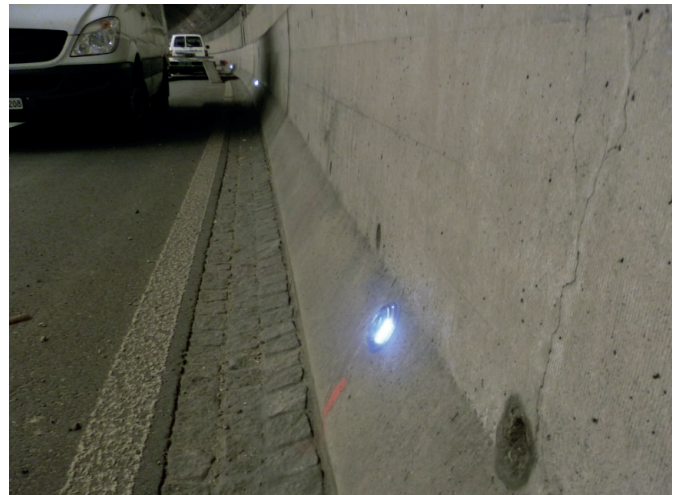
Tunnel Stephanshorn St. Gall
